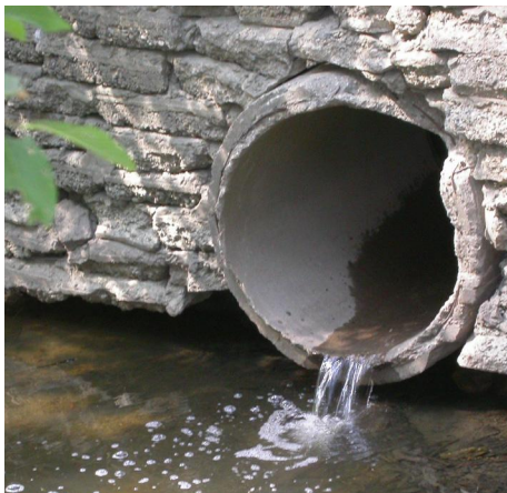
Of the 5,510 outfalls investigated, only 134 instances of illicit discharge were found between 2003 and 2008.
